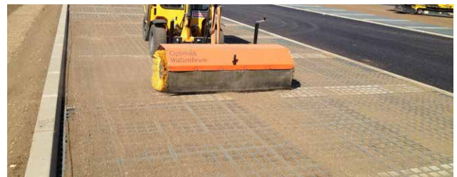
Produce the underfilling using a sweeper
