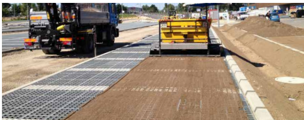
Insertion of the filling with a paver
