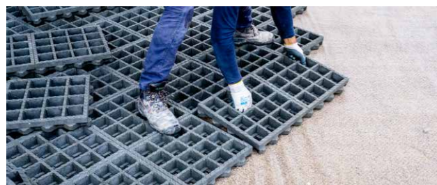
Laying of the TTE® elements on the fine matrix (installation aid).
